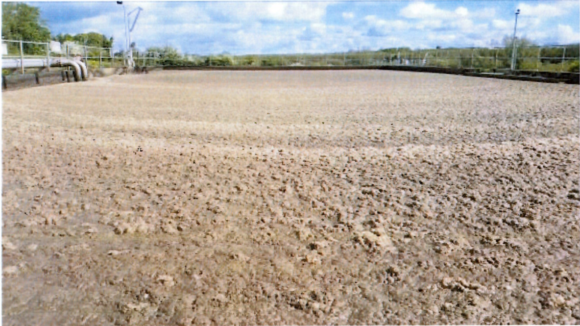
Photograph 1: Excessive foaming observed in aeration tank 1.
