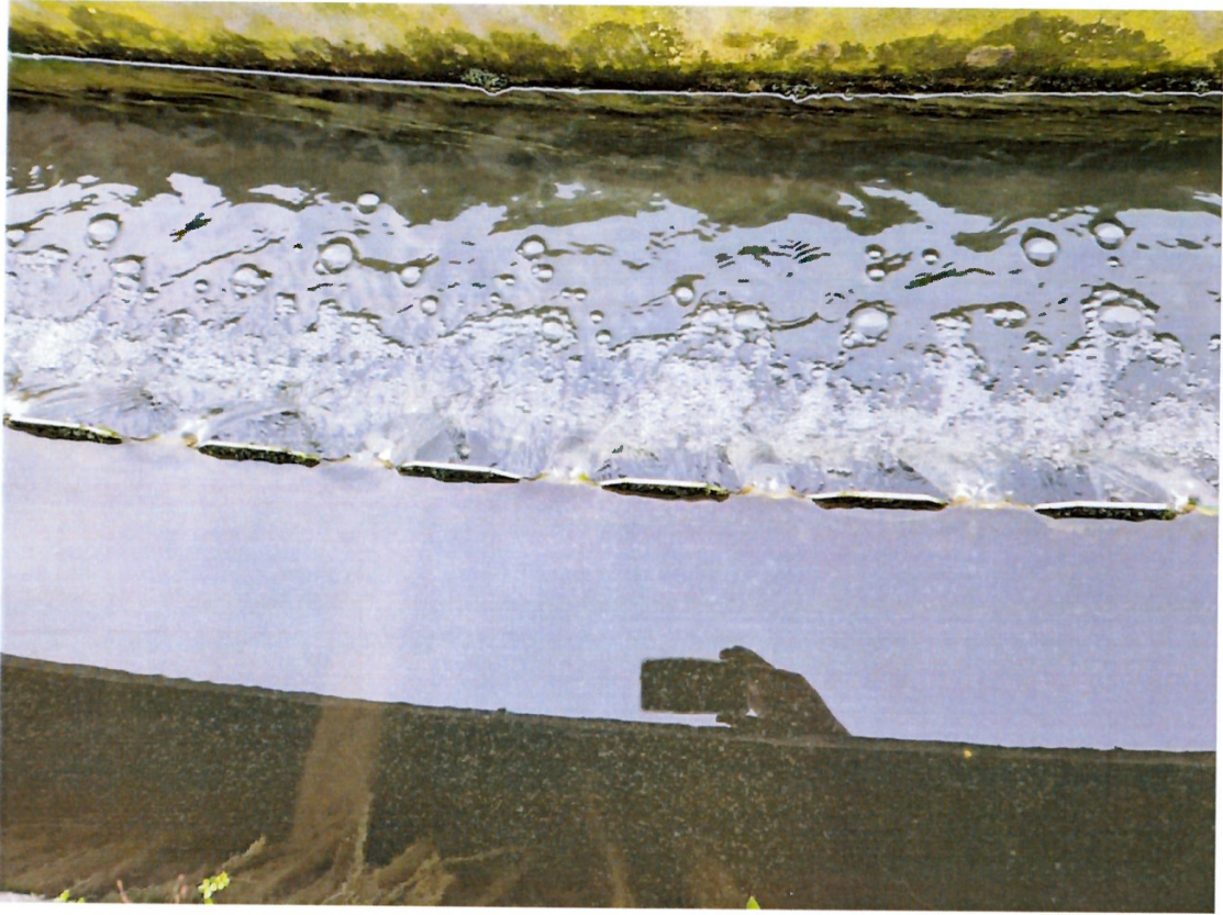
Photograph 3: View of Clarifier no. 1 at Ennis North Waste Water Treatment Plant (D0048-01)
